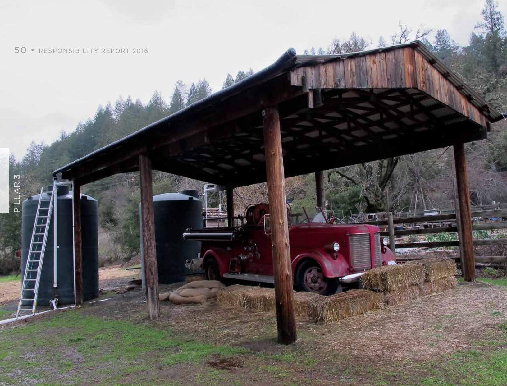
Tanks on rural properties adjacent to critical fish habitats capture rainwater for use during the summer months.
